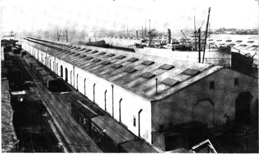
One of the Bush Piers, showing railroad tracks with cars waiting to receive cargoes to be transported direct from the ship
